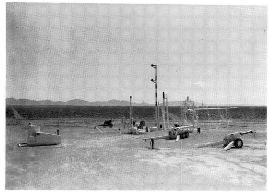
TEST AREA and overall view of the 155mm gun facility at Tonopah Test Range is shown in this photograph. The control bunker is in left foreground. The facility provides shock and acceleration testing for components encased in 155mm howitzer shells.
